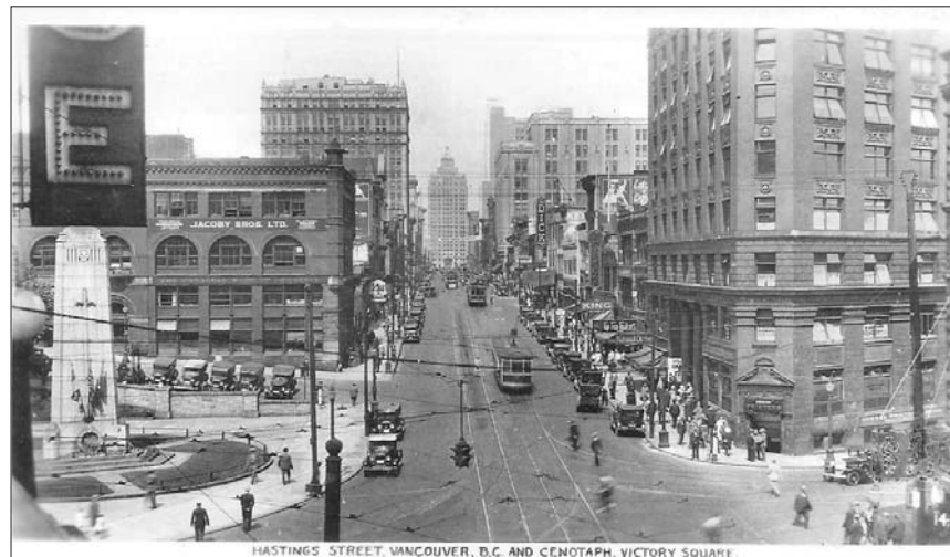
Fig. 2. Jacoby Brothers Ltd building beside Vancouver War Memorial on Hastings Street, 1922. Author's collection
