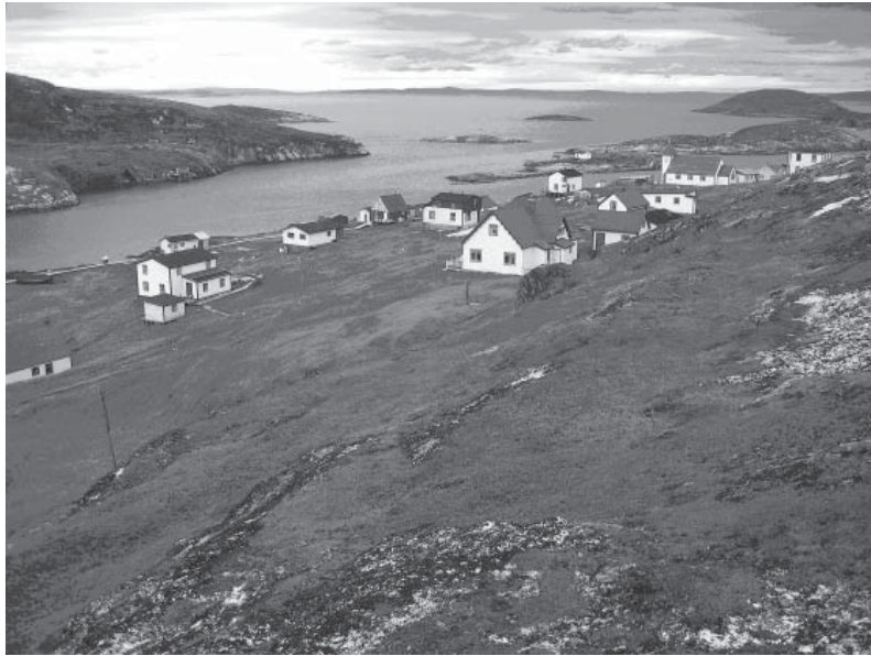
Figure 1. Looking northwest over the village of Battle Harbour, Labrador. Photo Michael Conzen.
